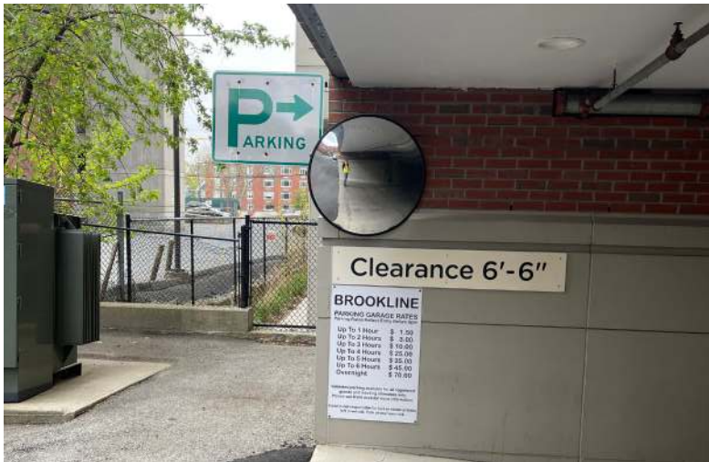
Without clear signage about who can park where, visitors may miss out on using facilities that are convenient to their destinations
